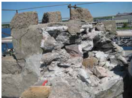
Fig. 2: Internal turret condition
