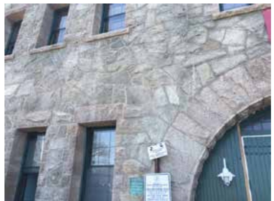
Fig. 11: Completed work before final wash-down
